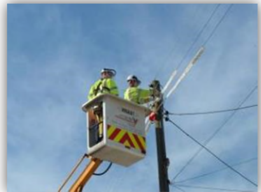
Fitting low energy LED lamps
